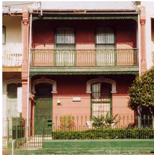
House on Wigram Street, Glebe Possibly one of Joseph Knox’s houses. Photo by Janet Fearby
