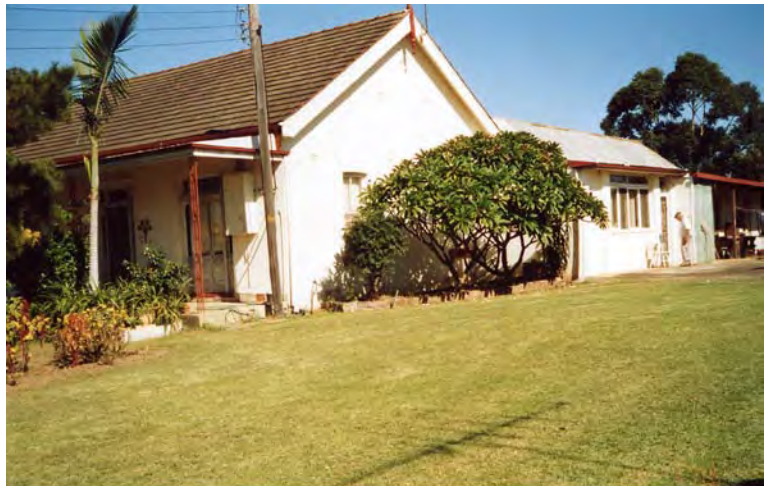
Joseph Knox's house, Montargis, Pendle Hill Build in the early 1890's
